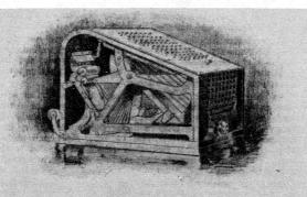
The First Model of an Adding Machine Made by Mr. Burroughs
